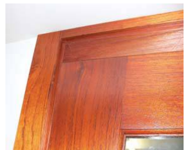
STEP 3 STANDARD DOOR WITH HEADBLOCK OVER
