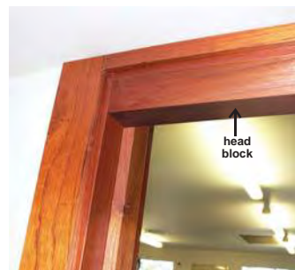
STEP 2 FRAME WITH HEADBLOCK INSTALLED
